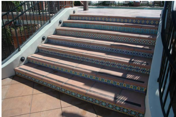
Hotel Roof Deck Access, Santa Barbara, CA
