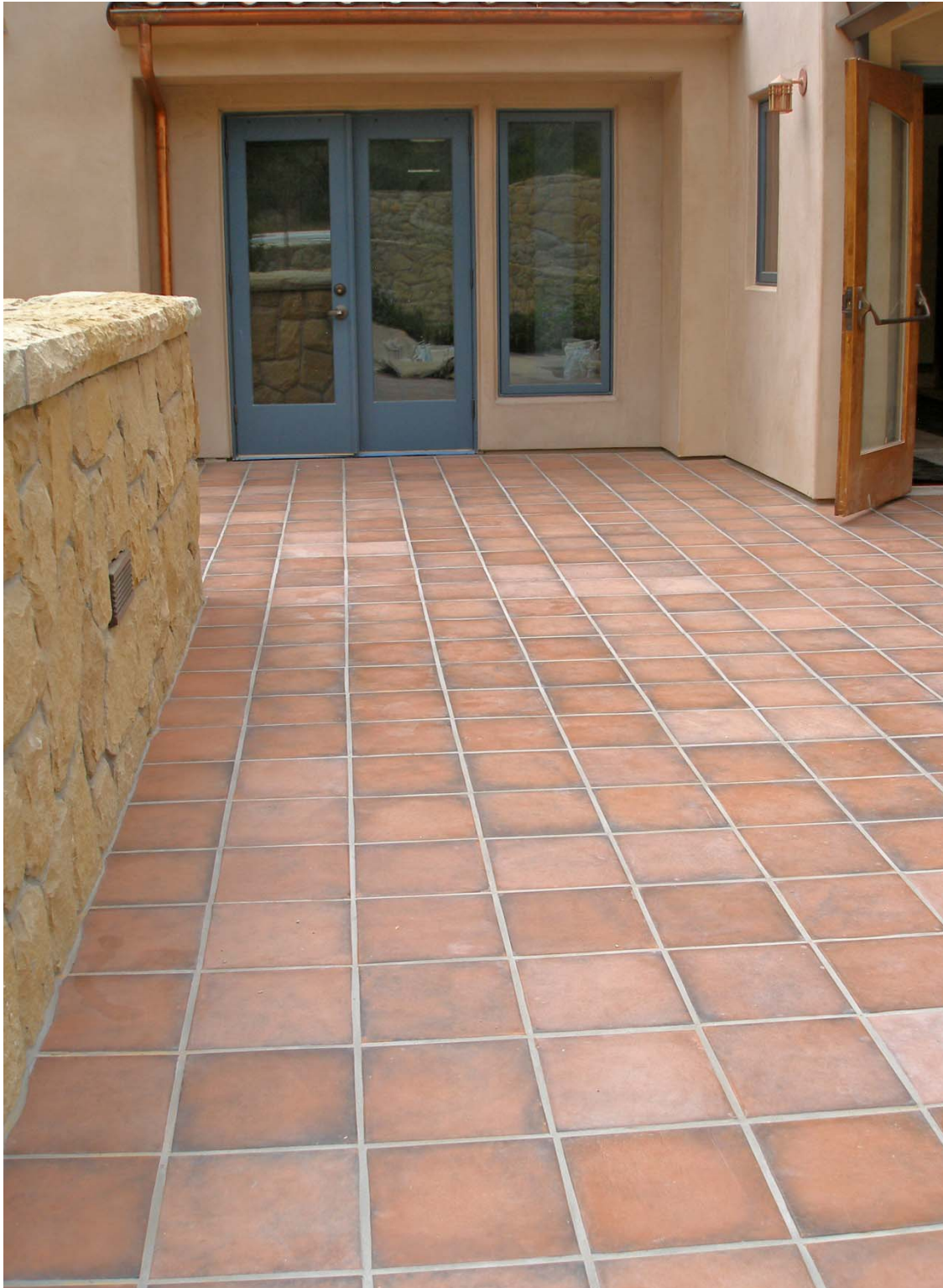
Orange Peel Eased Edge 12"x12" Mexican Terracotta, hospice facility, Santa Barbara, CA
